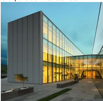
Phoenix Zeppelin Headquarter building is equipped with WAMAK heat-pumps
